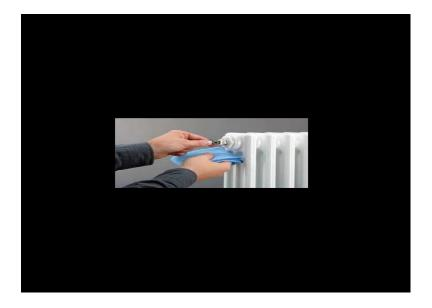
Does your heater not seem to heat right? Do you hear bubbling inside of it when it's turned on? Then you need to bleed the heater!
